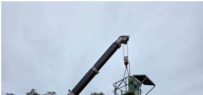
Tower head craned into place
