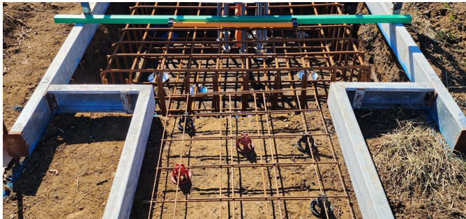
Foundation cage set out and checked before the pour
