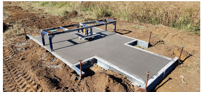
Finished slab, ready for the tower
