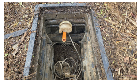
Sensor pit at the creek
