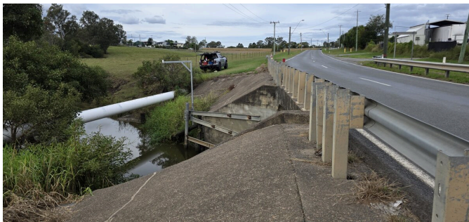
Culvert crossing on a busy road
